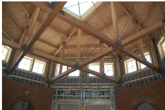
Inside the lobby area looking at the ceiling
